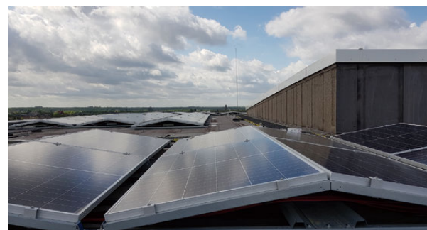
Solar panels at Canon Production Printing Netherlands
